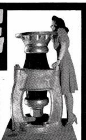
This giant base insulator supports one corner of the new WABC tower.
